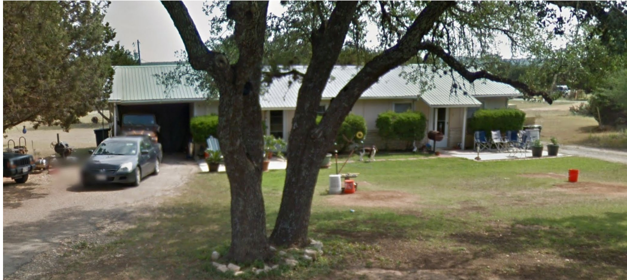
Exterior View of Existing Duplex
